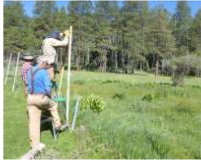
Removing and replacing old fence
